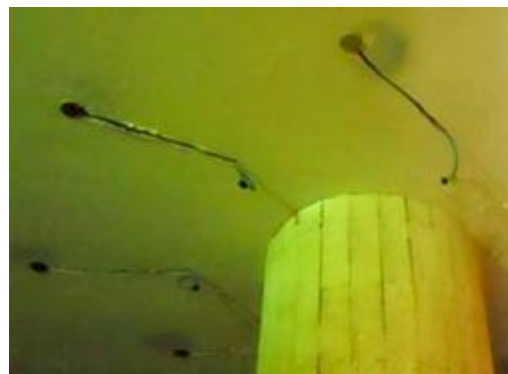
Furrows of the electrician after the plasterer did his job
